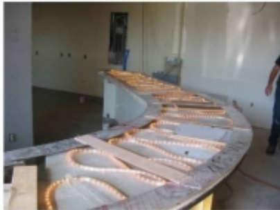
ABOVE LEFT- EXAMPLE OF A LIGHTED ONYX BAR TOP IN CONSTRUCTION, DESIGNED BY THE SCHIMBERG GROUP.
